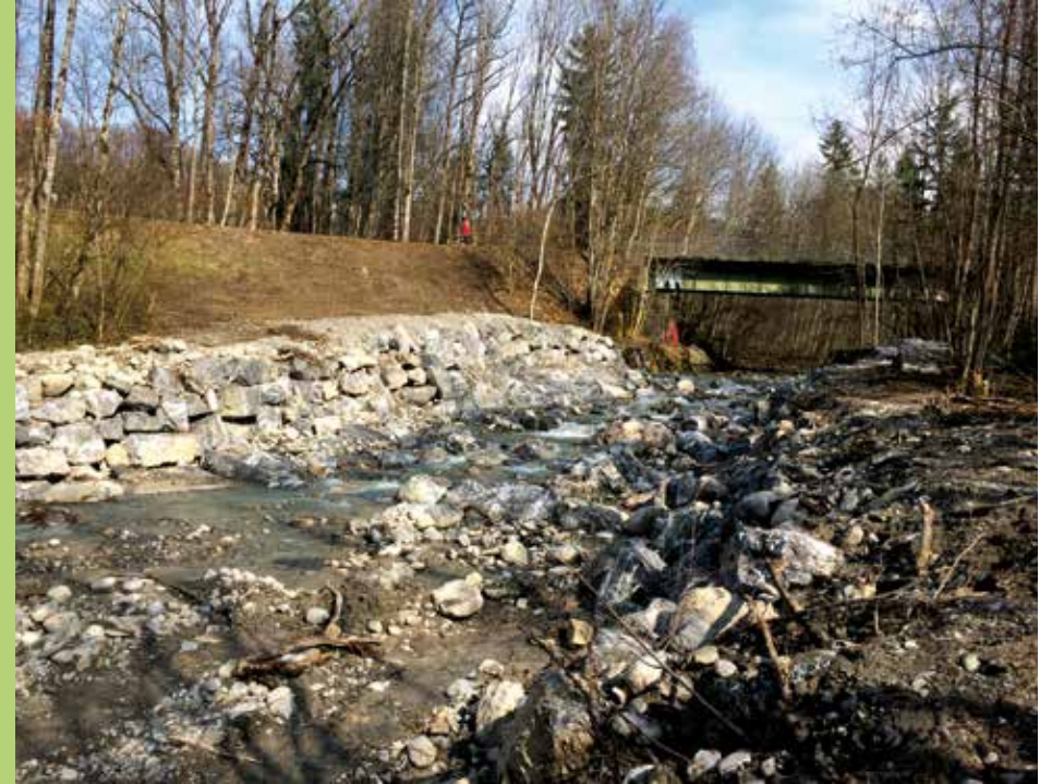
Fig. 9: Same location as picture 6, after renovation using a ramp stem.
