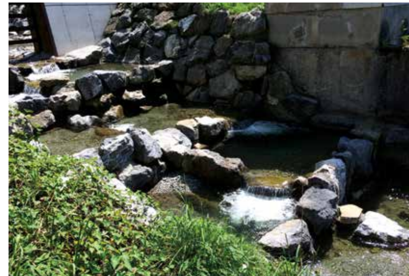
Fig. 4: Ramps instead of a dam torrent Steinebach
