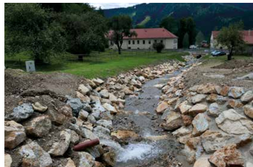
Fig. 2: Torrent Oberer Tollingbach before and after construction
