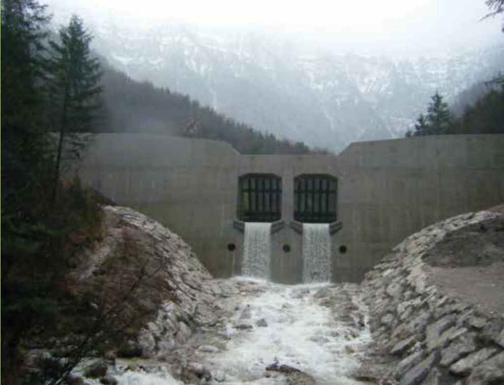
Fig. 8: Downstream view of the filtering dam
